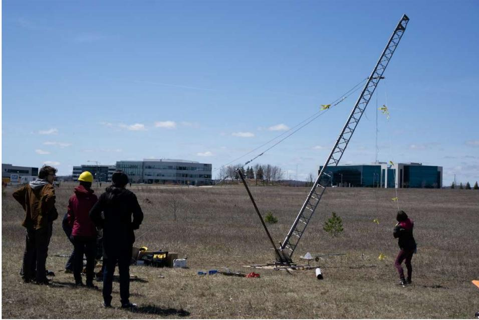
**Fig. 153 Raising the launch tower to a vertical position**
